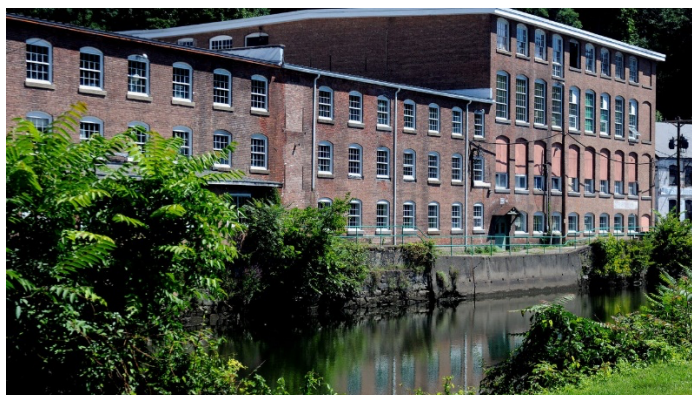
Figure 1: Building at the Bleachery
