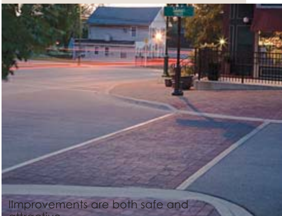
Corner bulb-outs and greening to narrow intersections
